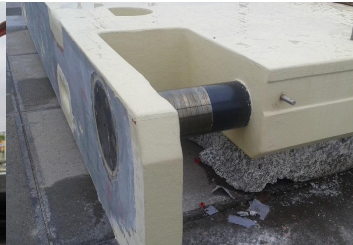
Hinge construction
